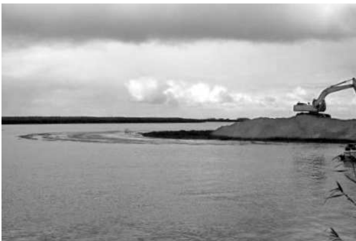
Constructing the "bund" at Narrung Narrows. March 2008 Lesley Fischer
