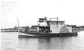
1930s The 'Tarella' side-paddle steamer took members of the River Murray Commission to the mouth to inspect proposed sites for barrages.
