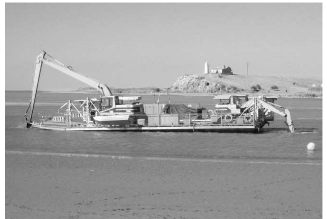
Dredging at Narrung, Lake Alexandrina side, using a ferry as a barge. 21 February 2009 Lesley Fischer
