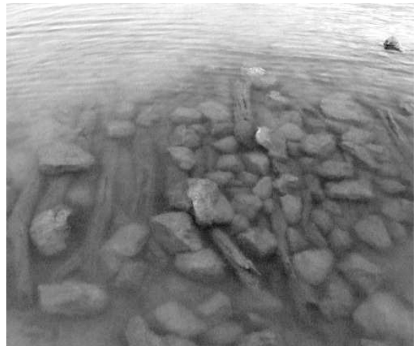
"Corduroy" and limestone ford across an ephemeral creek built on Yelland's farm c1870, seen here through shallow water in 2007. John Yelland
